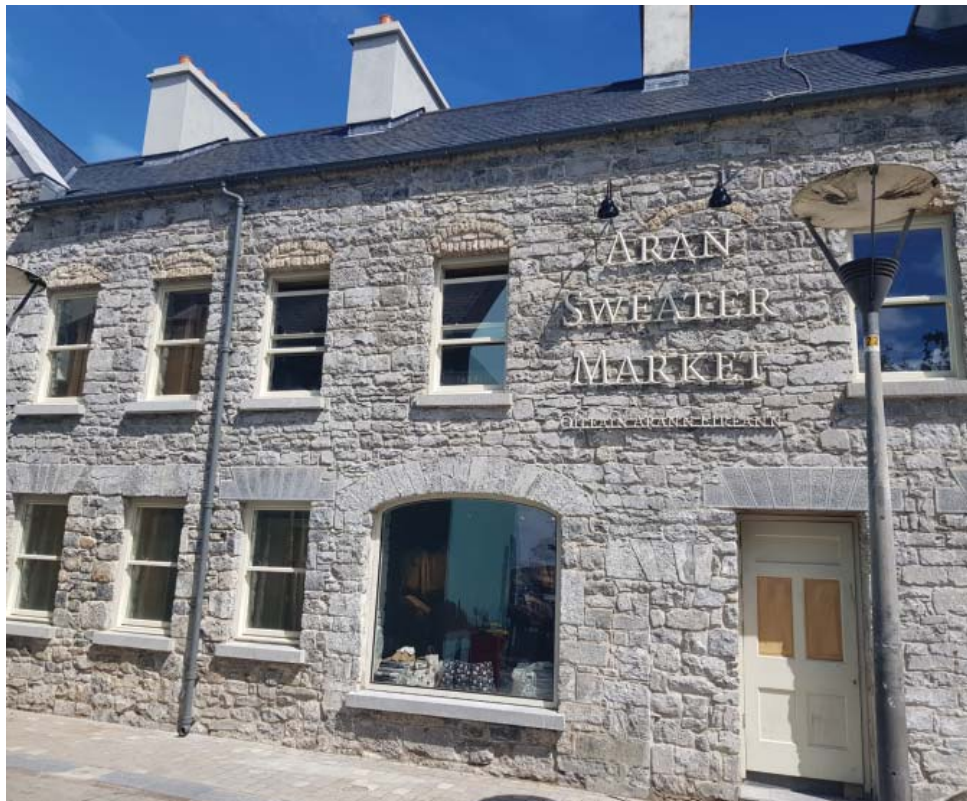
Fig. 44: The restored building now housing the Aran Sweater Market
