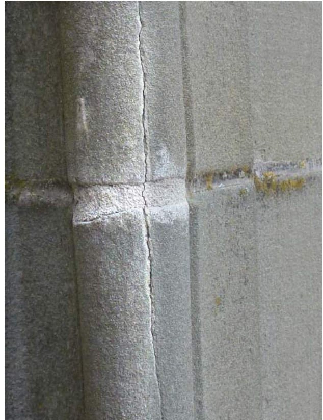
Fig. 4: Newly opened gaps in 2013
