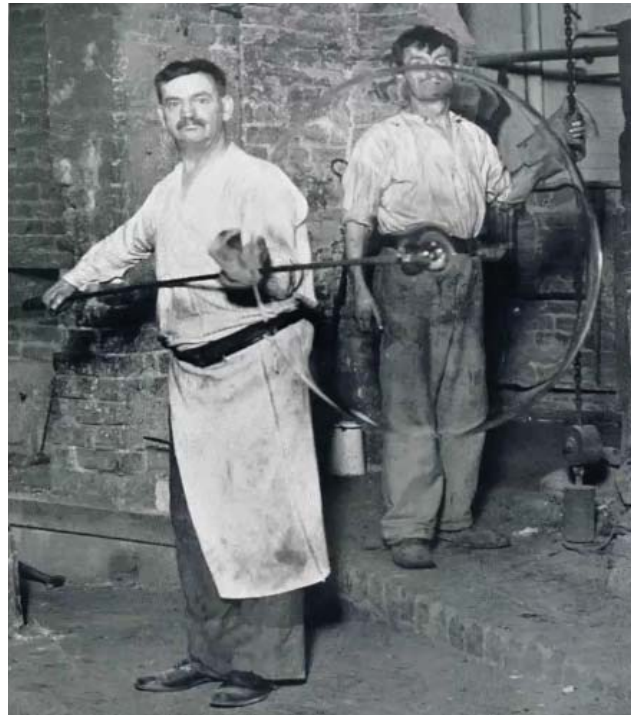
Fig. 6: Crown glass being spun by glass blower
