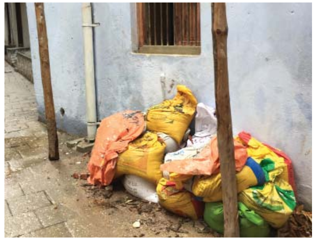
Image 8: Storage of bags with waste and contaminated building material against the historic wall (Beckett 2016)
