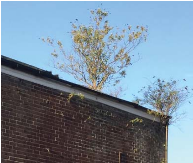
Image 5: Buddleia growing in rain gutter (Beckett 2020)
