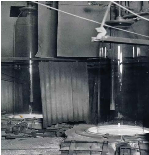
Fig. 10: The ‘improved cylinder method’, the large scale mechanization of the cylinder glass process
