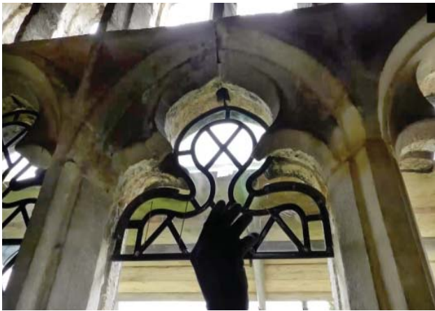
Fig. 27: Stained glass panels being inserted into the groove in the stonework
