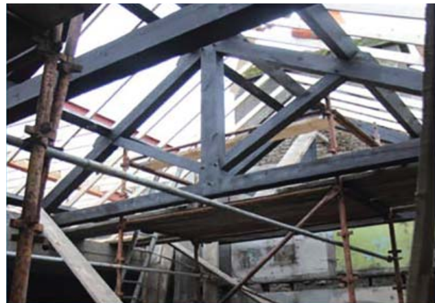
Fig. 37: The new roof being built on the concrete frame
