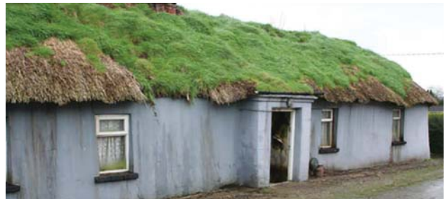
Fig. 10: Old thatched cottage in need of repair
