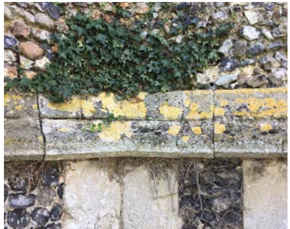
Image 38: The roots of Ivy an penetrate any voids and cause stress to the historic fabric (Beckett 2019)
