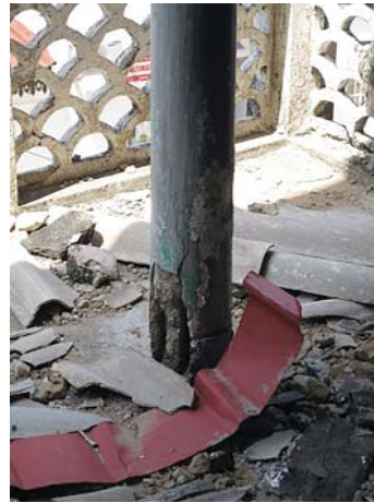
Image 7: Corrosion of reinforced early concrete pillars. (Beckett 2016)
