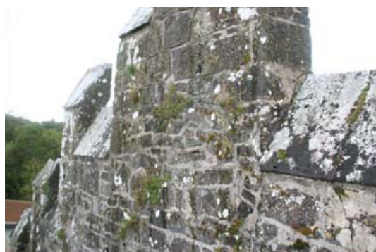
Fig. 26: Cement pointing done leading to stone damage
