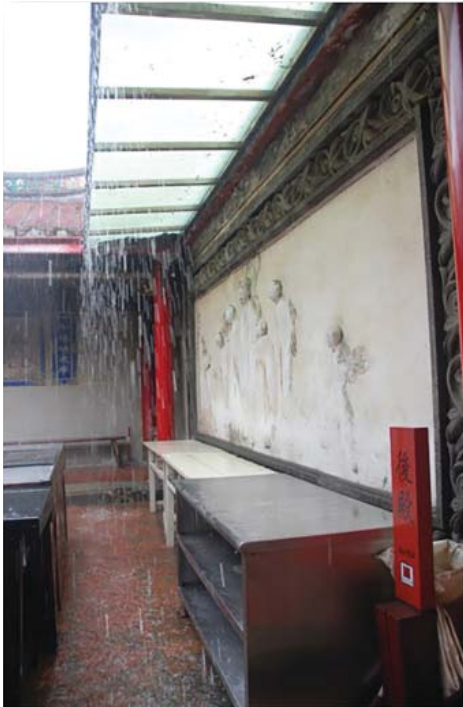
Image 32: Shuixian Temple, small. Protective temporary roof over the wall-painting stops direct rain. The later storage of the tables enables nevertheless the rain to bounce back onto the painting. (Beckett 2009)
