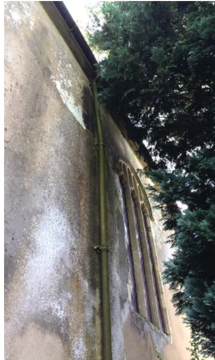
Image 14: Tree close to a historic building can hinder ventilation and cause mechanical damages (Beckett 2019)
