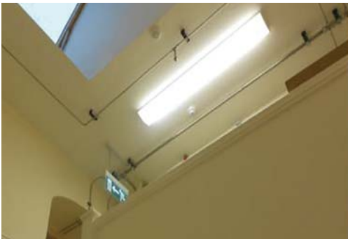
Fig. 28: Electrical fittings and fire safety equipment installed in traditional building
