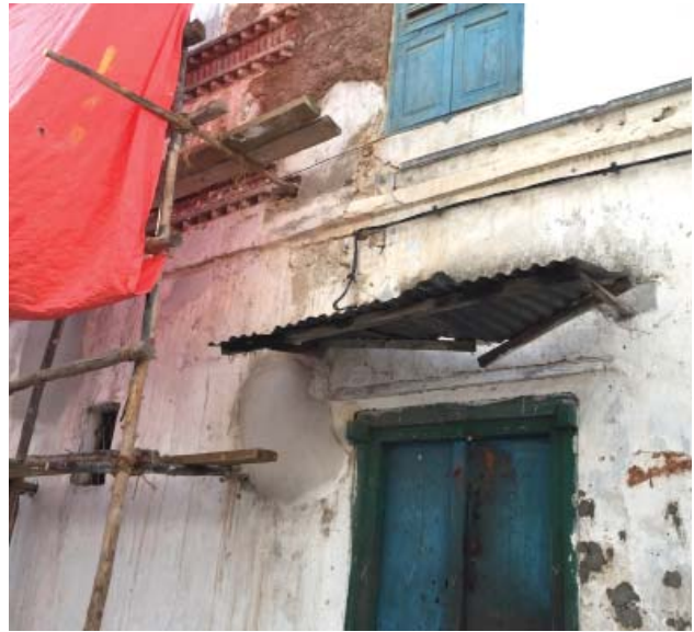
Image 10: Broken protective roof leads the water in the plaster of Hamamni Baths, Stone Town (Beckett 2016)
