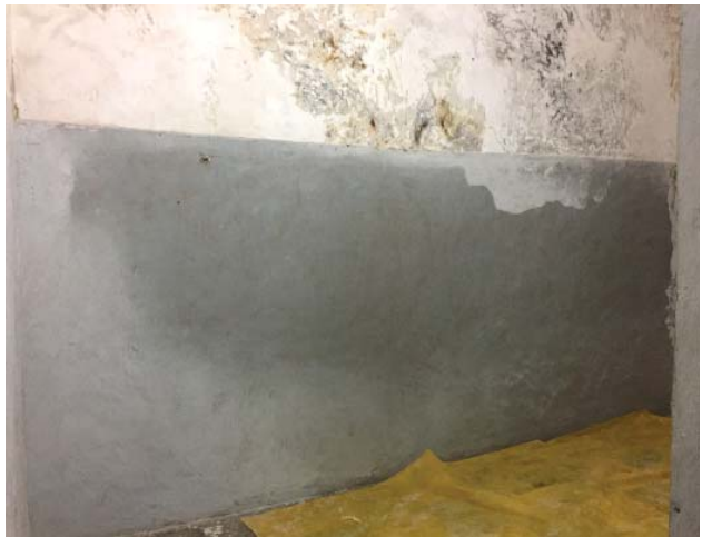
Image 29: Hamamni Baths, Interior. After rain the East wall is getting in one area. (Beckett 2016)
