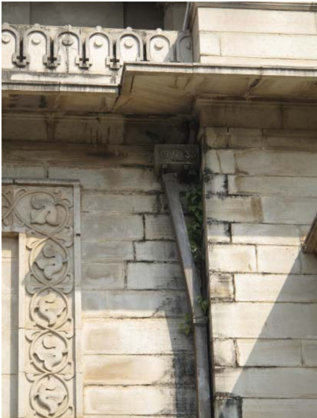
Image 24: Kirti Mandir: Cast iron downpipe. The biological growth indicates that water leaks out. Birds, here a pigeon is resting in the hoppers and contaminate the water and block the hopper.
