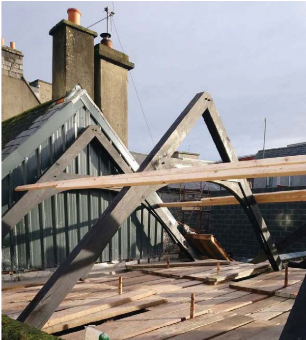
Fig. 39: Medieval style roof trusses were designed and constructed within the 15th century building section
