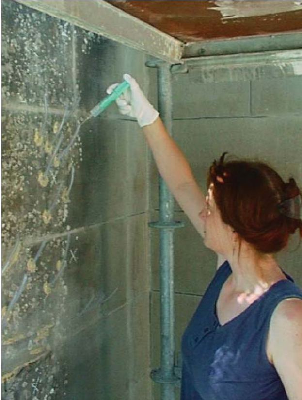
Fig. 3: Grouting around 2000
