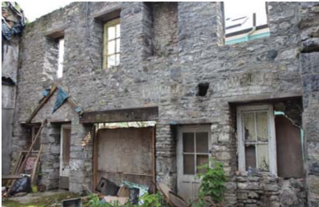
Fig. 31: The interiors of the property with the missing roof, windows and other architectural elements
