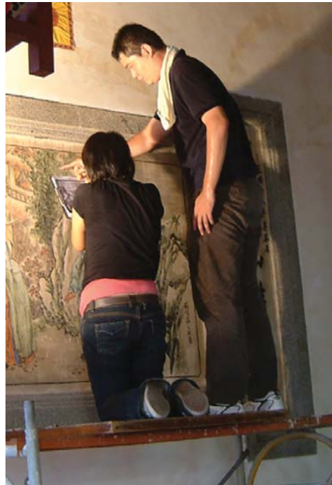
Image 34: Shuixian Temple in Beigang. Students from the TNNUA are carrying out regular monitoring and maintenance (Beckett 2010)
