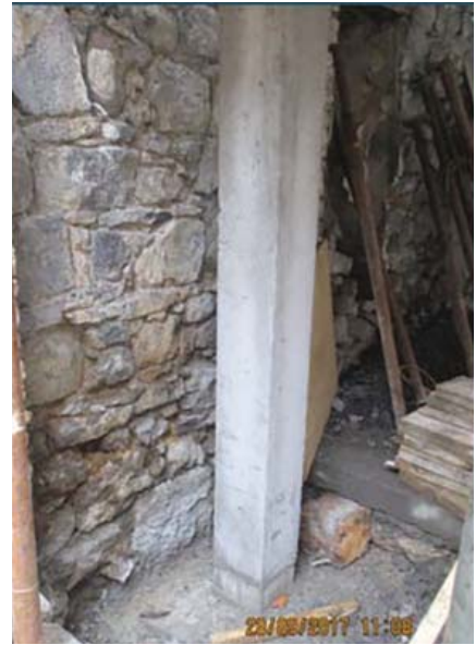
Fig. 35: Concrete column to carry the main structure
