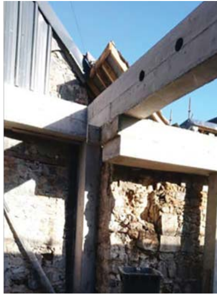
Fig. 34: Detail of the concrete frame designed to support the building
