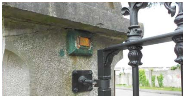
Fig. 23: A new gate installed in place of an old gate that could have been restored
