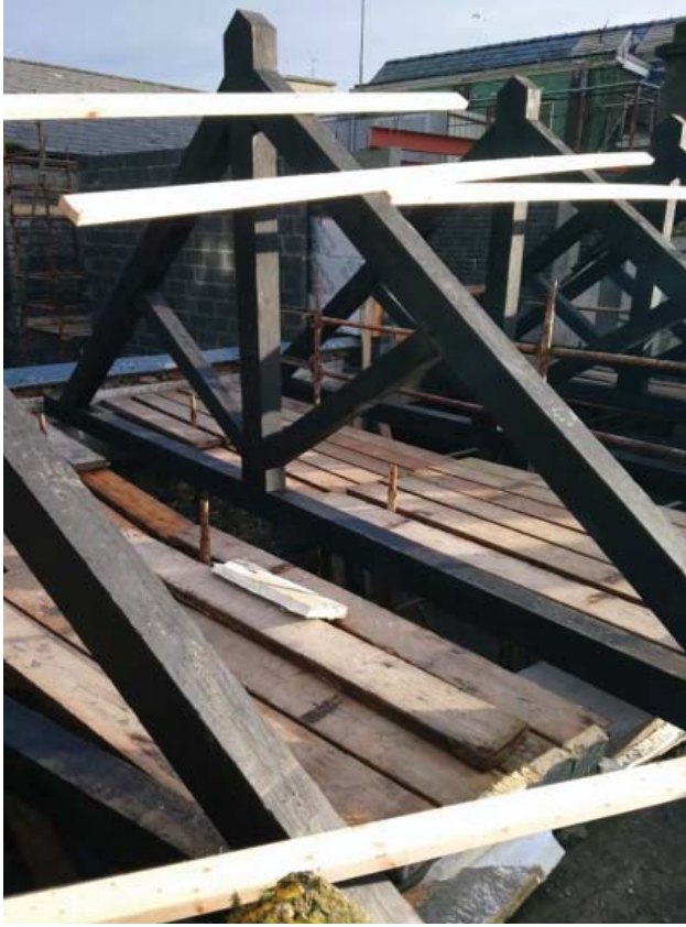
Fig. 38: 'King post' truss roof within the 19th century section of the building
