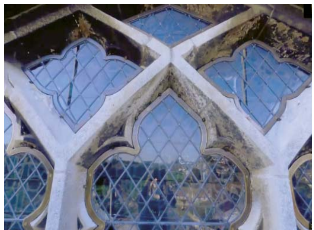
Fig. 30: EPG system where 3D scans were taken to cut bronze frames for external glazing
