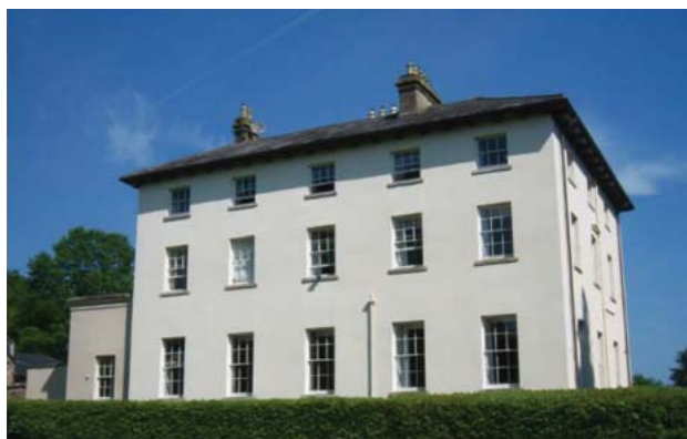
Fig. 24: A building with OPC plaster rendering
