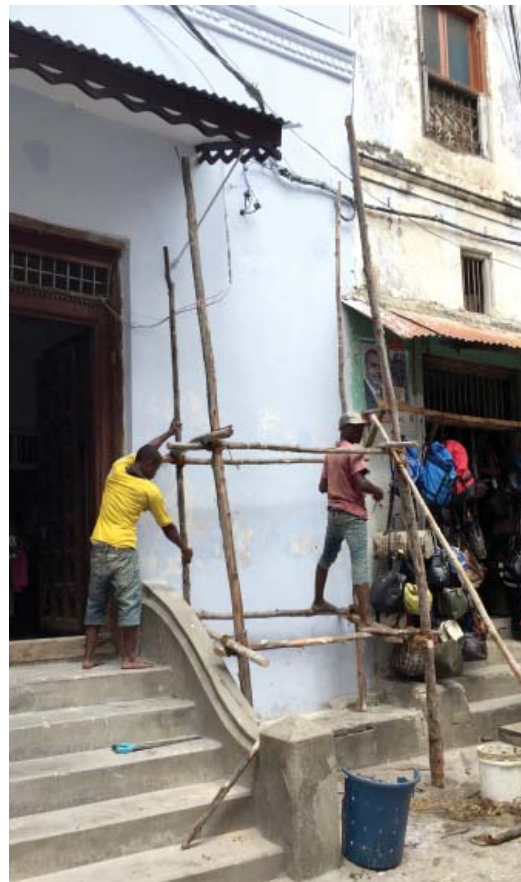
Image 11: Broken protective roof leads the water in the plaster of the “Upendo House”, Stone Town and activates soluble salts. (Beckett 2016)
