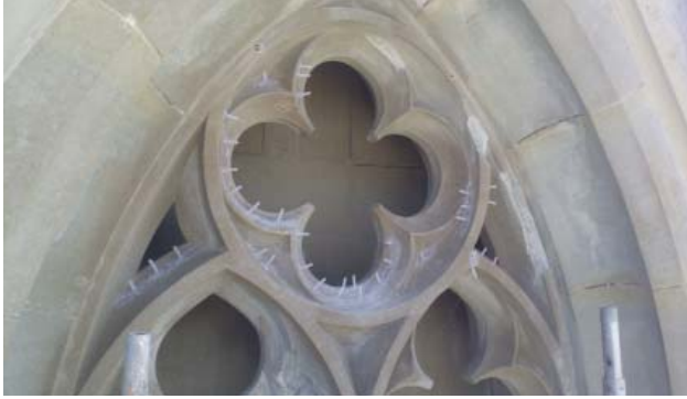
Fig. 5: Preparation for consolidation and grouting
