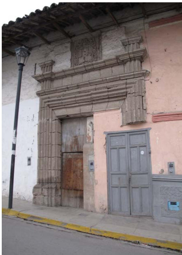
Fig. 5: Inappropriate opening (Photo: Norma Barbacci)
