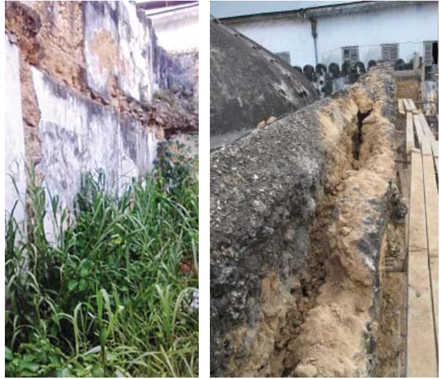
(Left) Image 27: Hamamni Baths, East wall exterior before clearing, waste and contaminated standing earth (Beckett 2016)
