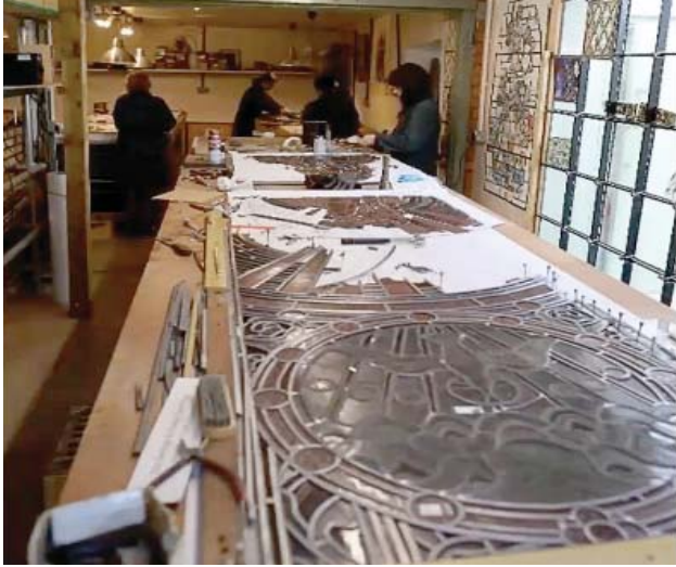
Fig. 26: Re-leading of the Great East Window panel
