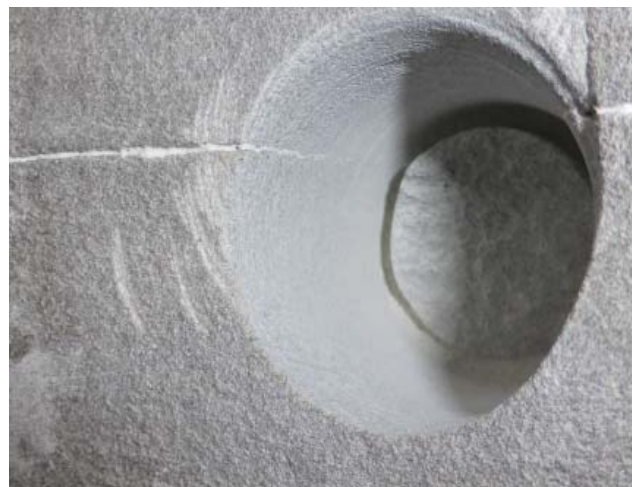
Fig. 6: Gap refilled with silicic-stone-adhesive. Diameter of hole 28 mm.
