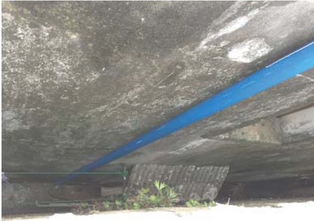
Image 30: Hamamni Baths. The downpipe from the neighbouring house drains the water into the east wall of the Hamamni Baths. (Beckett 2016)
