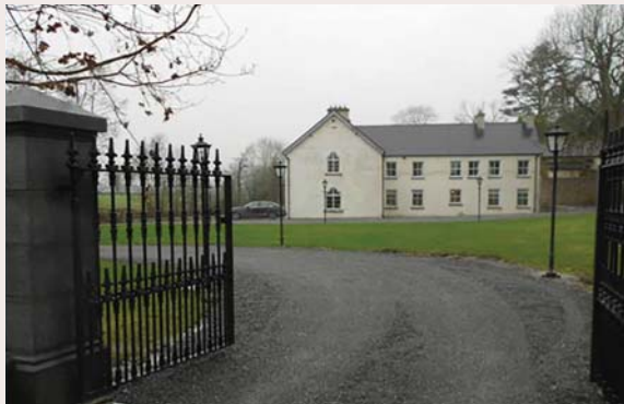
Fig. 8: The building and the surroundings after restoration
