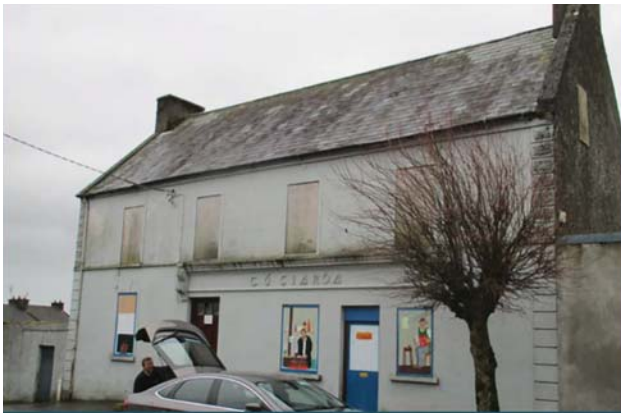
Fig. 5: An example of a family home with a shop that is no longer economical so the house is left boarded up to decay
