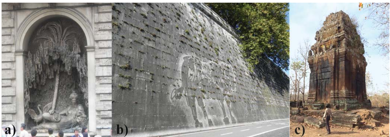
Fig. 7: The different origin for the black/grey patina. a) The four fountain "Giunone" (Rome): car pollution; b) Tiber embankment (Rome): biological colonisation; c) Khmau temple (Cambodia): geological processes
