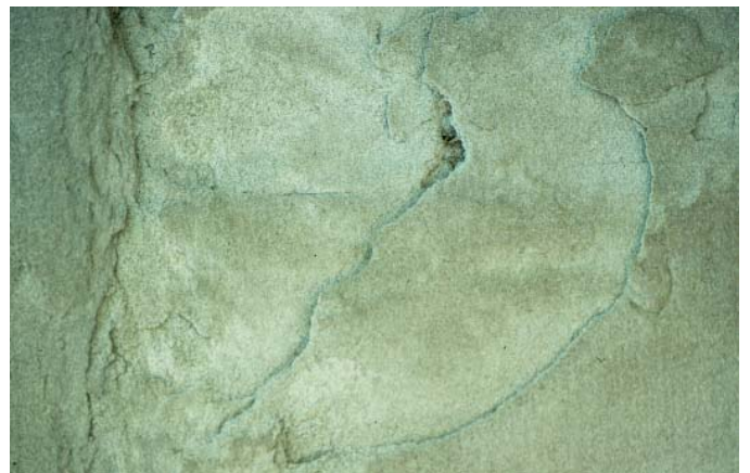
Fig. 2: Multiple layers of delamination in 1998
