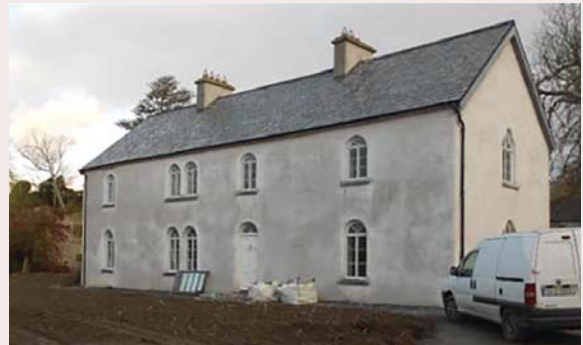
Fig. 7: The building during restoration
