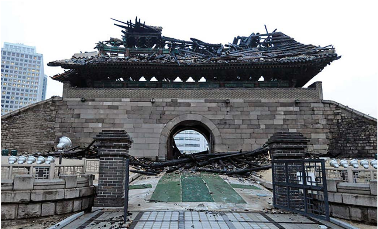
Fig. 8: Sungnyemun after the 2008 fire
