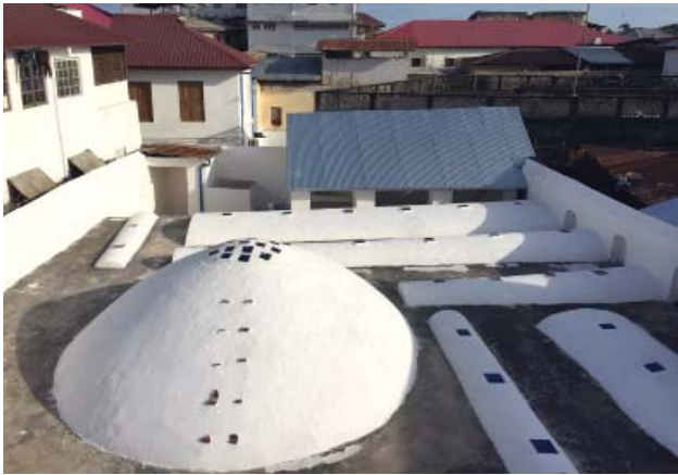
Image 26: Hamamni Persian Baths roof area after restoration (Beckett 2016)
