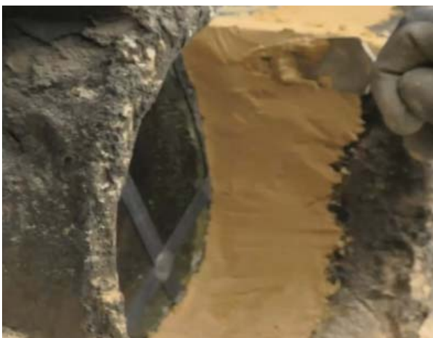
Fig. 28: Application of lime mortar for fixing panels in stonework
