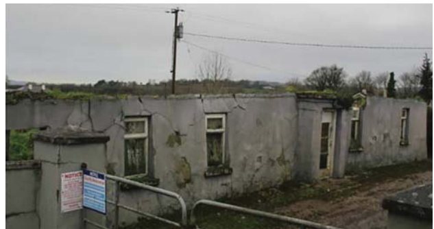
Fig. 11: The abandoned building with structural damage and loss of thatching.
