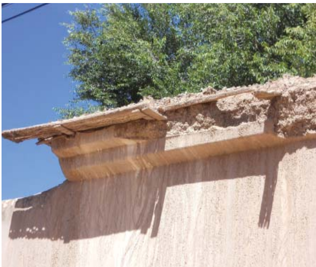
Fig. 2: Adobe cornice damaged by moisture (Photo: Marcelo Magadán)
