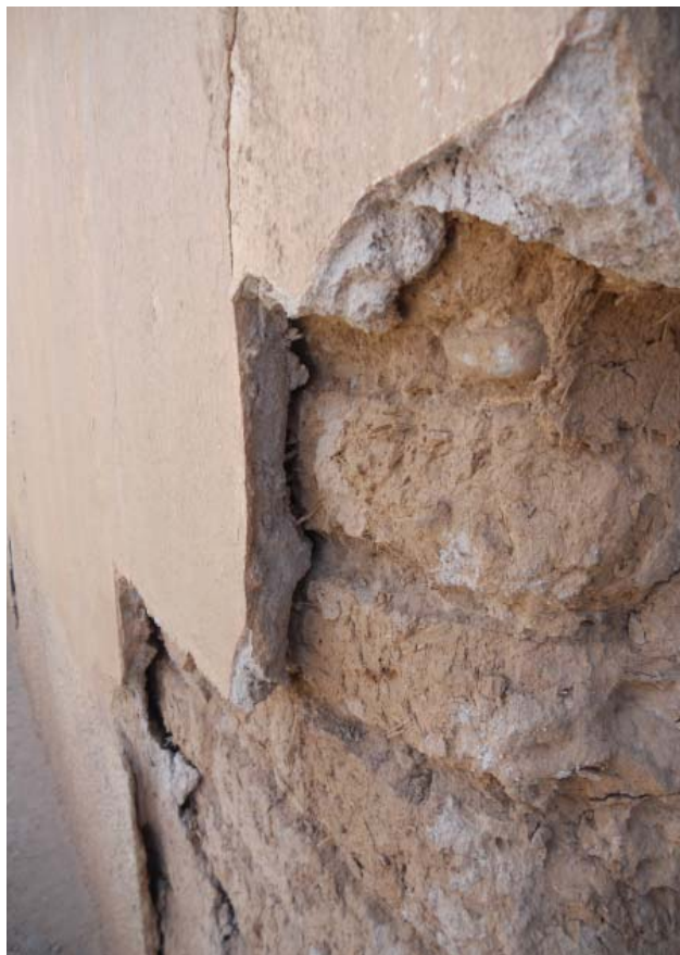
Fig. 4: Cement coating on adobe wall (Photo: Marcelo Magadán)
