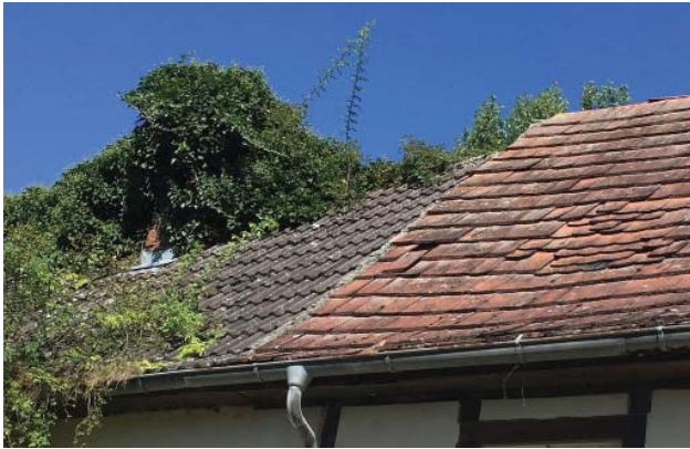
Image 4: Slipped, displaced and lost roof tiles (Beckett 2020)
