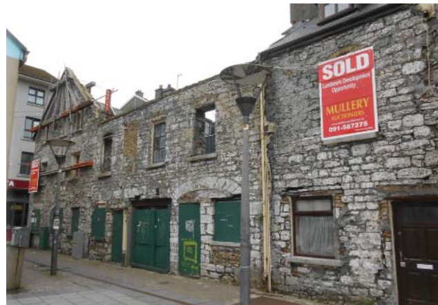
Fig. 30: Quay Street property before restoration
