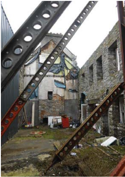
Fig. 33: All the internal walls had been demolished
