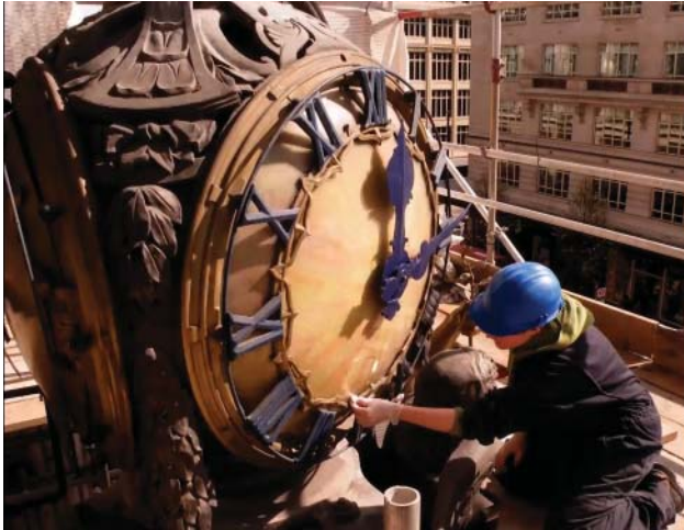
Fig. 5: Repair work being undertaken on a clock belonging to Selfridges department store
