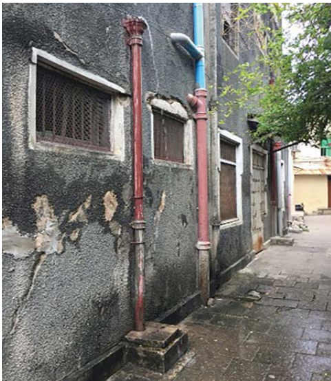
Image 6: Defect, overflowing downpipe (Beckett 2016)
