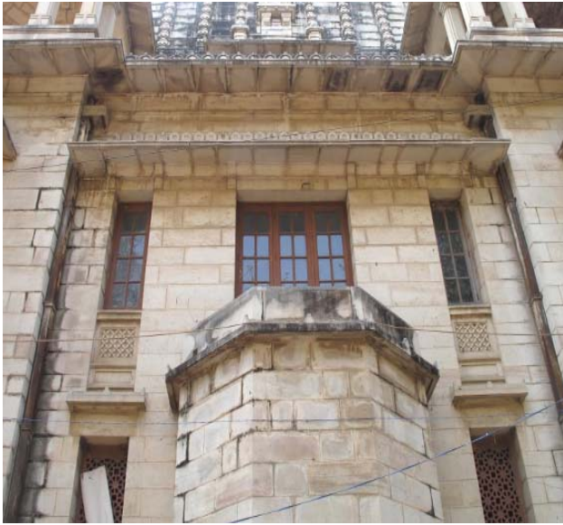
Image 23: Kirti Mandir: On the exterior there are two historic cast iron downpipes on the areas where the wallpaintings inside show defects.
