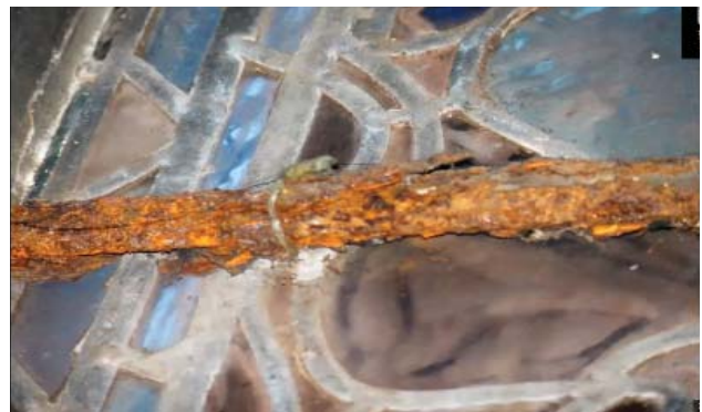
Fig. 33: Highly damaged tie bar
