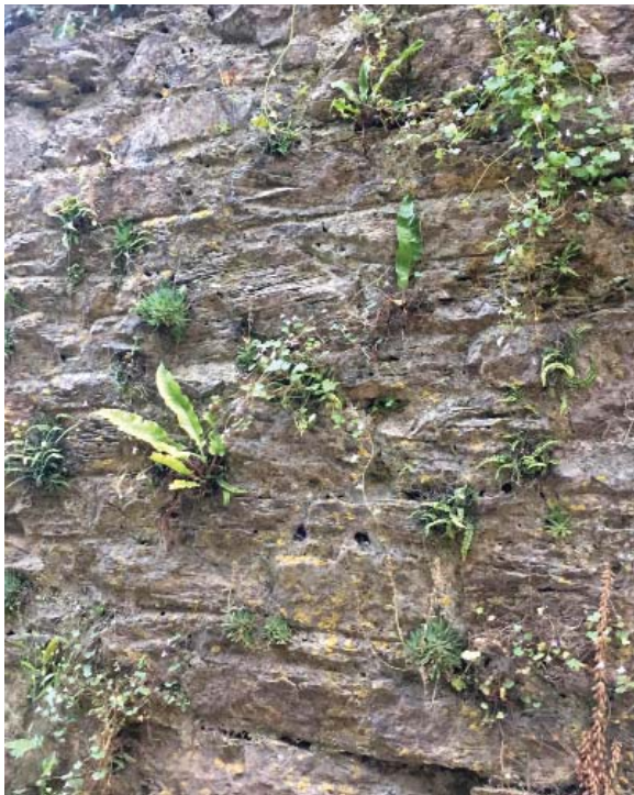
Image 36: Historic Stone wall with a variety of protective and harmful biological growth. (Beckett 2020)
