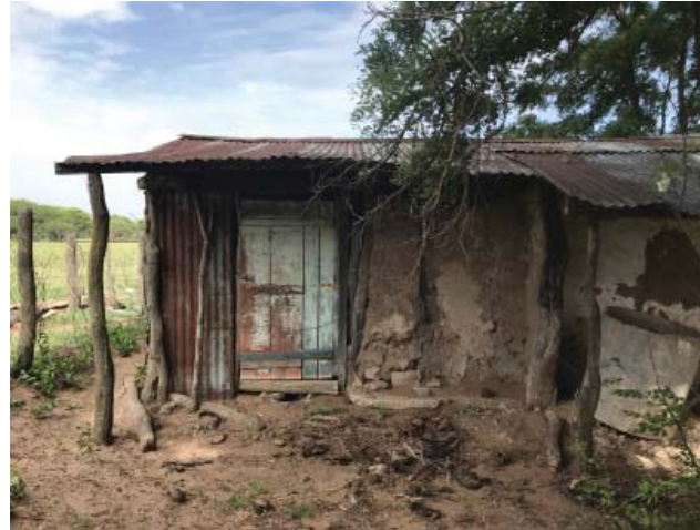
Fig. 3: Poorly maintained adobe (Photo: Kevin Gartner)
